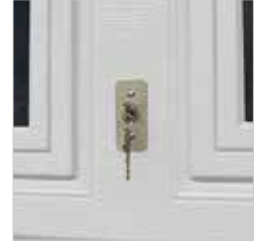
Vault Release Allows you to open and close the door during power outage.
